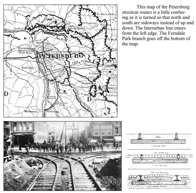
Streetcar tracks were laid in the same way as railroad tracks. Steel rails were spiked to wood ties. These were below the street level. The cavity was filled so that the top of the tracks were flush with the street. This prevented people from tripping on them.
